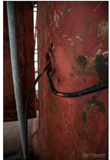
Images 81, 82 and 83: previous arrangement of cables in lantern room, going through vents to the exterior, and loose cables exiting vent on the outside
