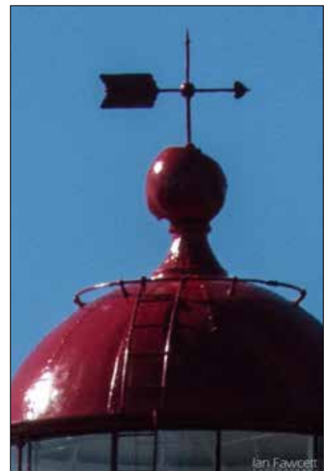
Image 63 and 64 (bottom centre and right): weather vane restored and reassembled atop lantern room
