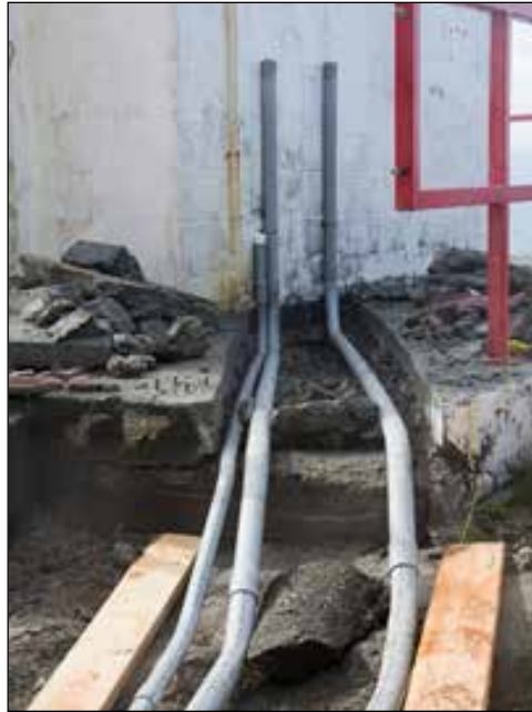
Image 27 (top left): forms for concrete conduit cover
