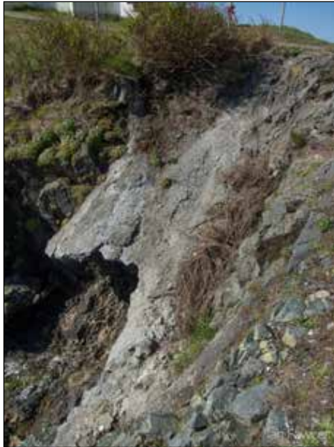
Image 3 (top left): erosion on the east side of the causeway
