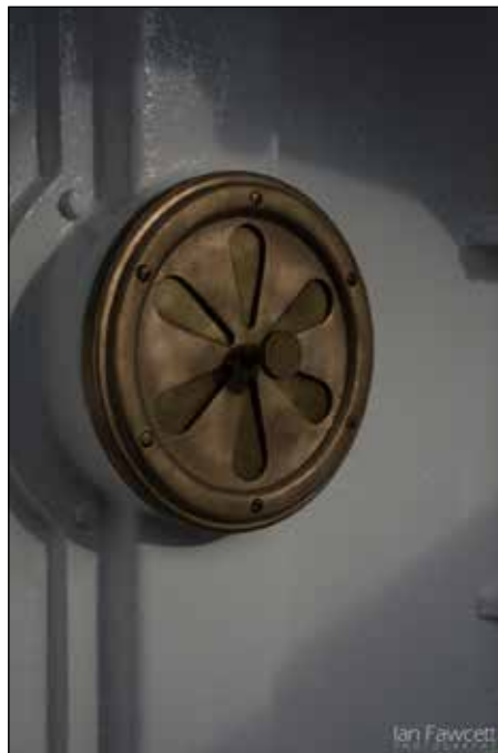
Image 78 (top left) and 75 (previous page): show vents in original condition
