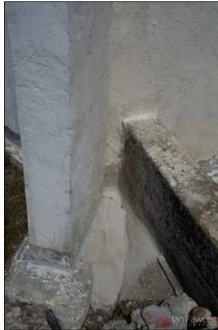
Images 98 and 99 (top row): excavation to address leakage issue - compound patches are points of water ingress
