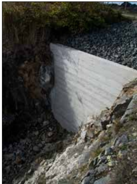
Image 6 (bottom left): reinforced retaining wall, with aggregate fill on east side of causeway
