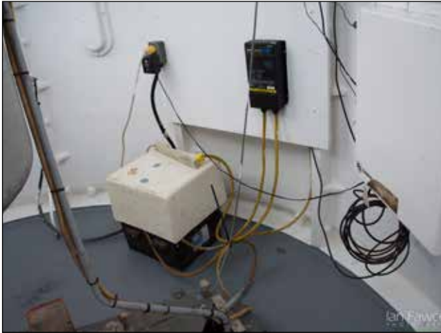
Image 84(left): showing cleanup of cables in lantern room
