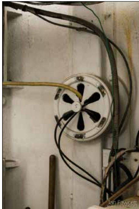
Images 81, 82 and 83: previous arrangement of cables in lantern room, going through vents to the exterior, and loose cables exiting vent on the outside
