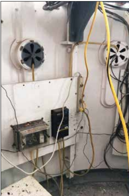
Images 81, 82 and 83: previous arrangement of cables in lantern room, going through vents to the exterior, and loose cables exiting vent on the outside
