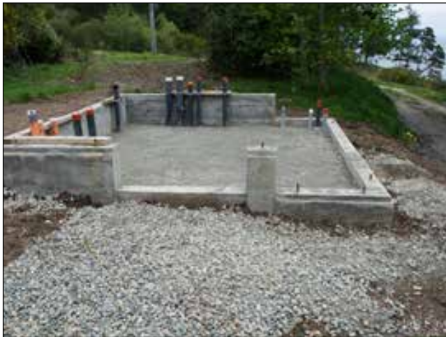
Image 17 (top left): excavation and foundation forms
