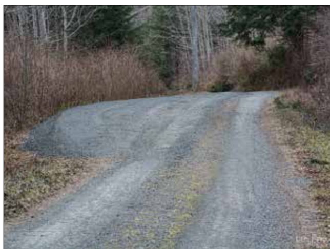
Image 144 (left): original road condition, with vehicle turnout (passing area) under development
