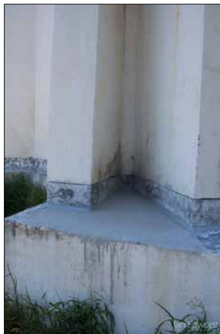
Images 100 and 101 (bottom row): water-proofing around base to protect from splash-back
